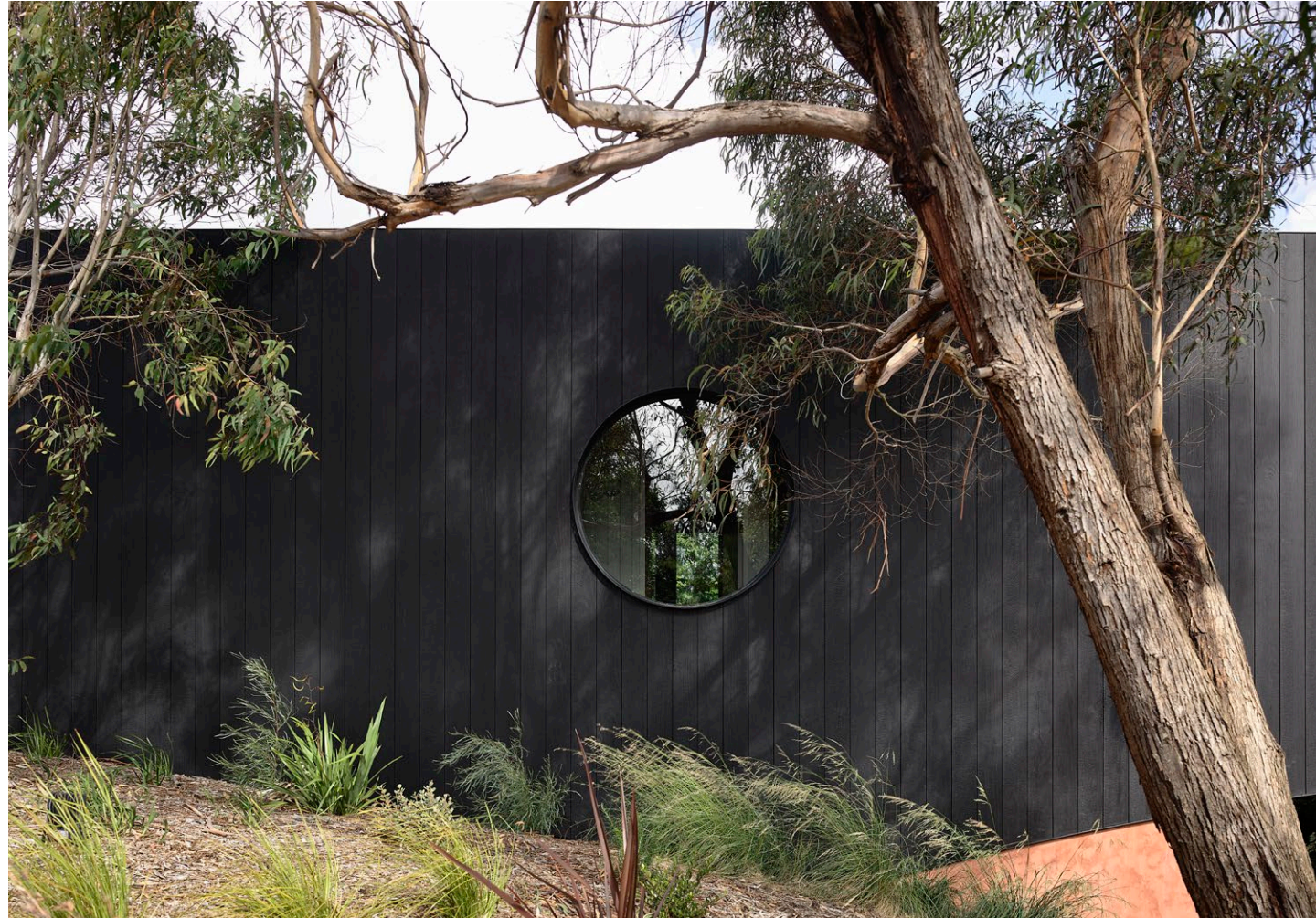
The exterior shell is formed from shou sugi ban charred timber and is interrupted by a small circular opening characteristic of Kennedy Nolan's work.
