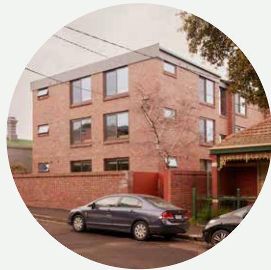
The south-facing façade of Wilam Ngarrang from the street.
